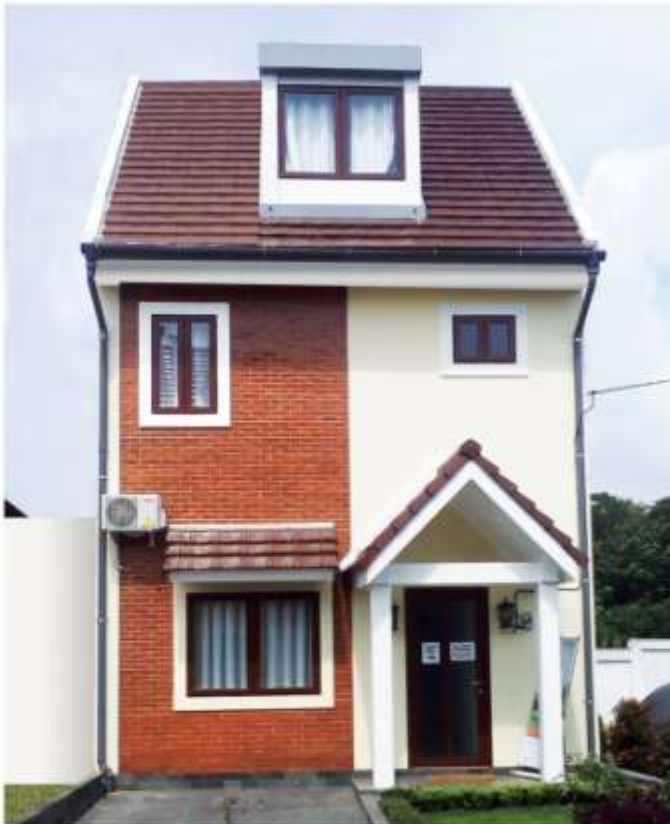
Pintu (Frame) & Jendela uPVC Finishing Hot Stamp Mahogany Brown + Kaca 5 mm.
